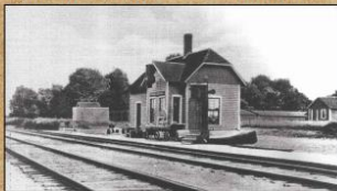
The Congamond Rail Station is shown in the L.J. Richards map of 1894, as being located about one-half mile north of Lake Road (now called Congamond Road). A long siding could accommodate 50 rail cars at a time to take patrons back to the cities after a day's outing at the lakes.
